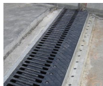
Sliding finger joints
