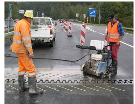
Cutting of slits at a 45° angle to the driving direction
